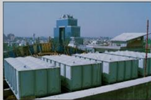
70 KL, 56 KL 2x42 KL for raw and drinking water at a Shopping Complex
