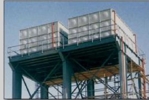
3m. Deep 2x72 KL tanks for soft water at a Milk dairy in Dubai.
