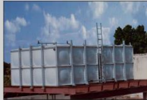
2x24 KL tank for Soft Water at a Soft drink Plant
