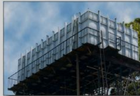
2.5m. Deep 180 KL tank for Drinking Water at a Residential Colony
